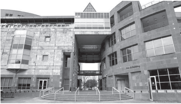
Frio St. Building, UTSA Downtown Campus.
