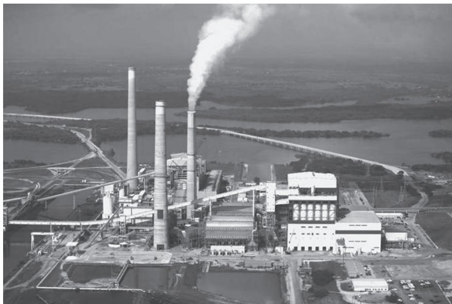
CPS Energy’s four coal plants including Spruce 2 (center smoke stack closest to camera) which was completed on Calaveras Lake on Sept. 15, 2010. Photo by Lisa Krantz, Staff / SA Express-News
