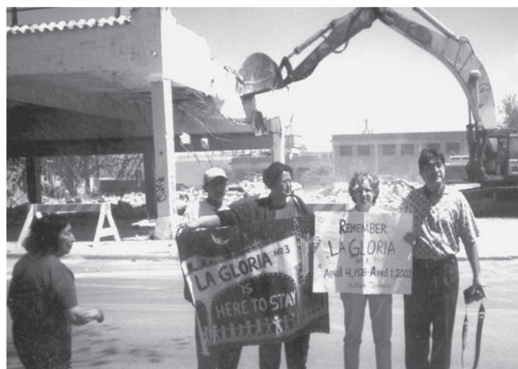
Community protestors at the demolition. Remember La Gloria April 4, 1928 to April 1, 2002.
